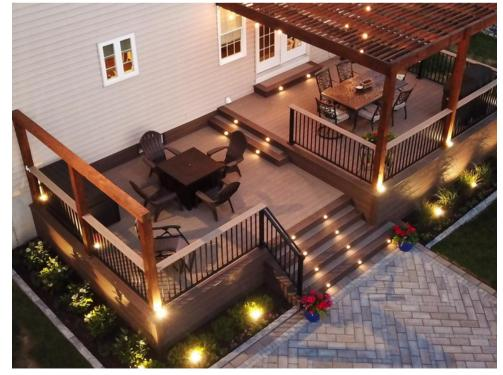
PROJECT BY BY PREMIER OUTDOOR LIVING VOYAGE DECKING IN MESA AND KHAYA WITH CONTEMPORARY RAIL IN TEXTURED BLACK WITH SECONDARY HANDRAIL, DECK BOARD RAILING CONNECTOR AND LOW-VOLTAGE RECESSED LIGHTING.
