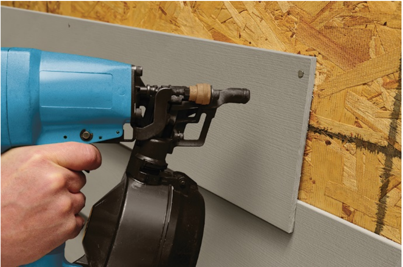
FIGURE 2—EOTEK SIDING INSTALLATION
