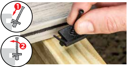
1. Wedge into groove
