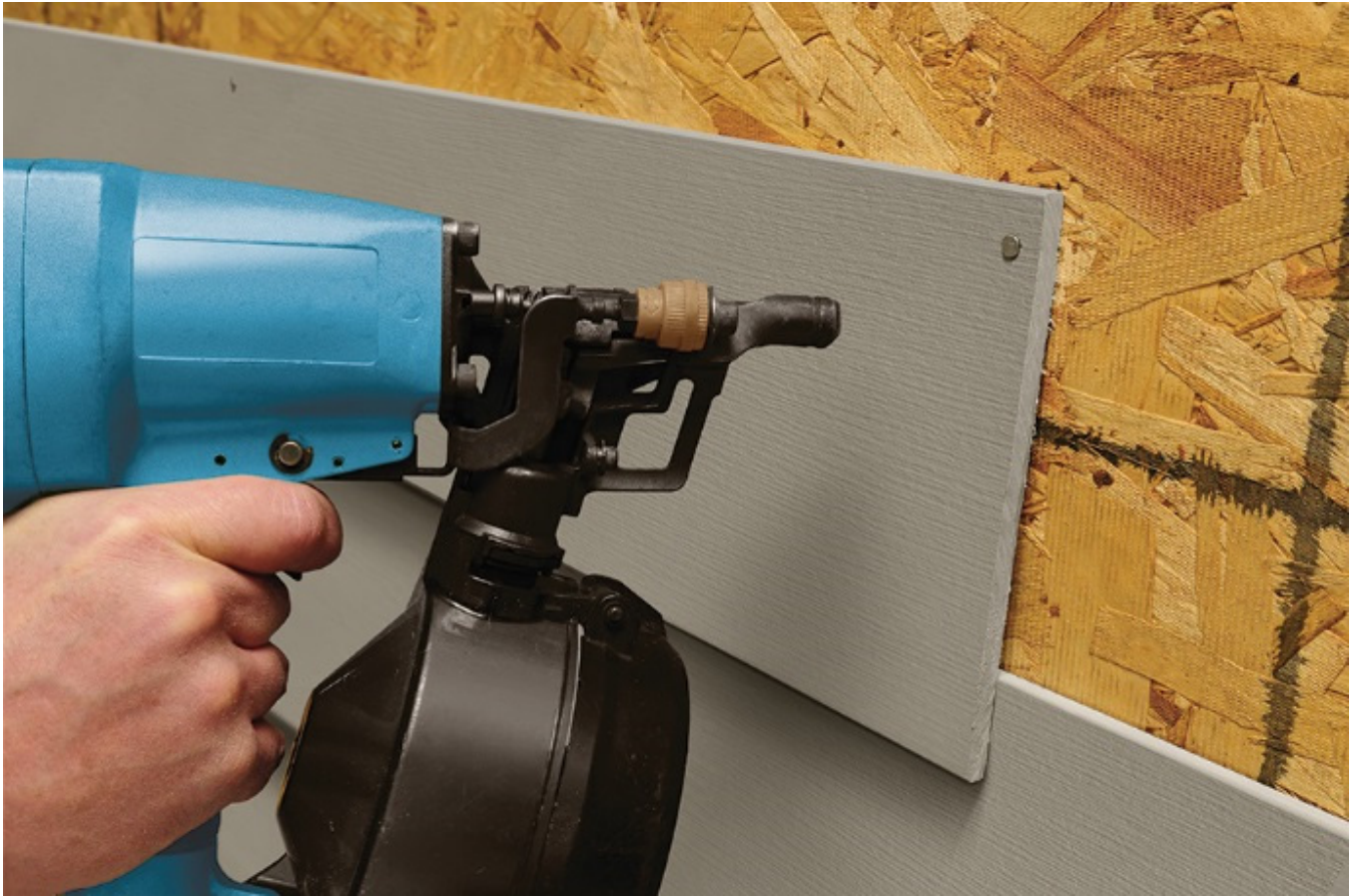
FIGURE 2—EOTEK SIDING INSTALLATION
